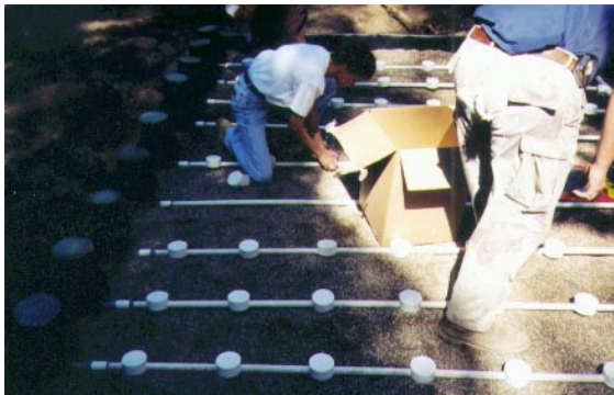
Figure 9. Intermittent Sand Filter
