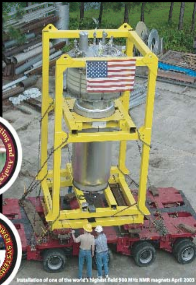
Installation of one of the world's highest field 900 MHz NMR magnets April 2003
